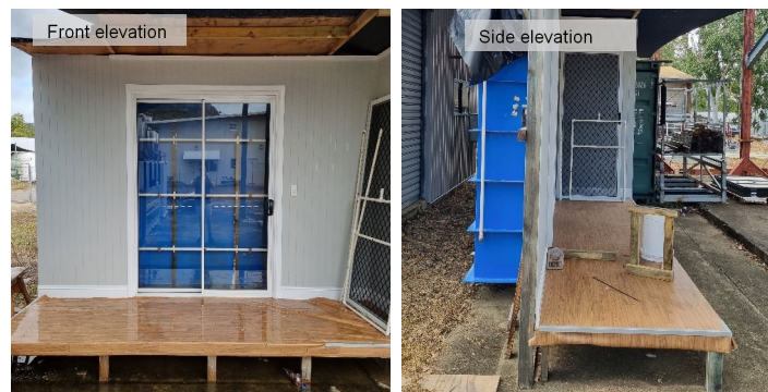
Figure 1. Wind-driven rain simulator test apparatus, C2 sliding glass door installed,
